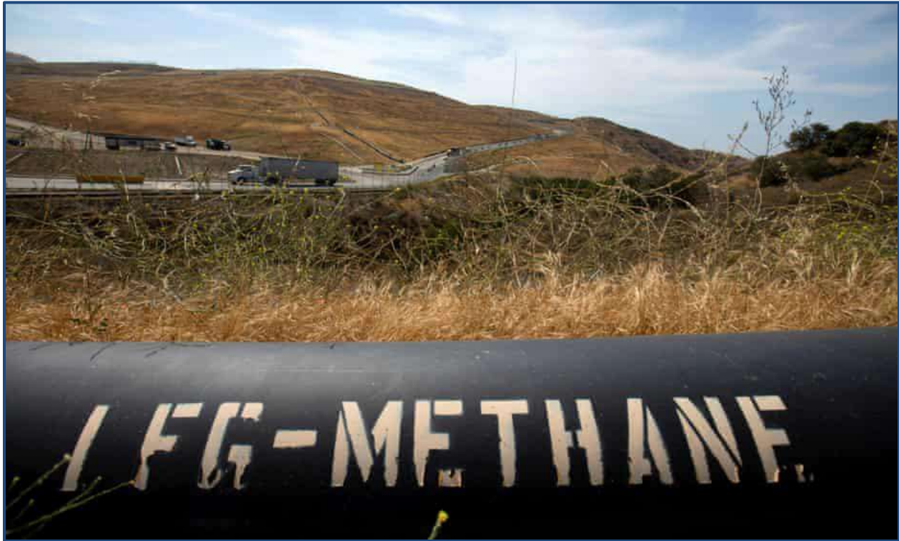
A pipeline that moves methane from a landfill to an onsite power plant in Irvine, California
