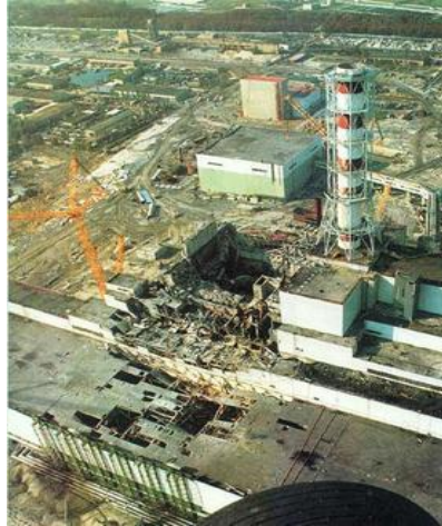
The nuclear reactor after the disaster. Reactor 4 (center). Turbine building (lower left). Reactor 3 (center right).
