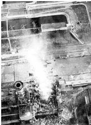
Aerial view of the damaged core on 3 May 1986. Roof of the turbine hall is damaged (image center). Roof of the adjacent reactor 3 (image lower left) shows minor fire damage.
