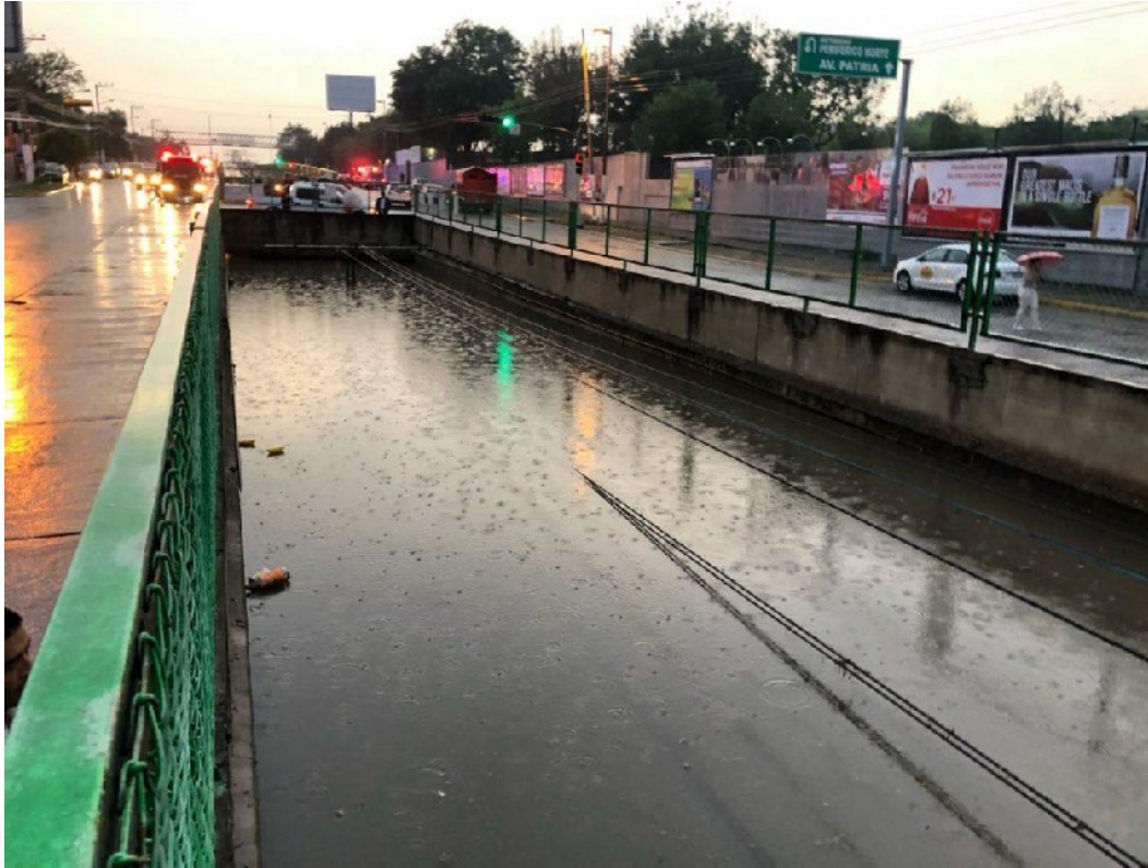
Flooded railway in Guadalajara, Jalisco, Mexico, 10 June 2018. Photo: Protection Civil Jalisco
