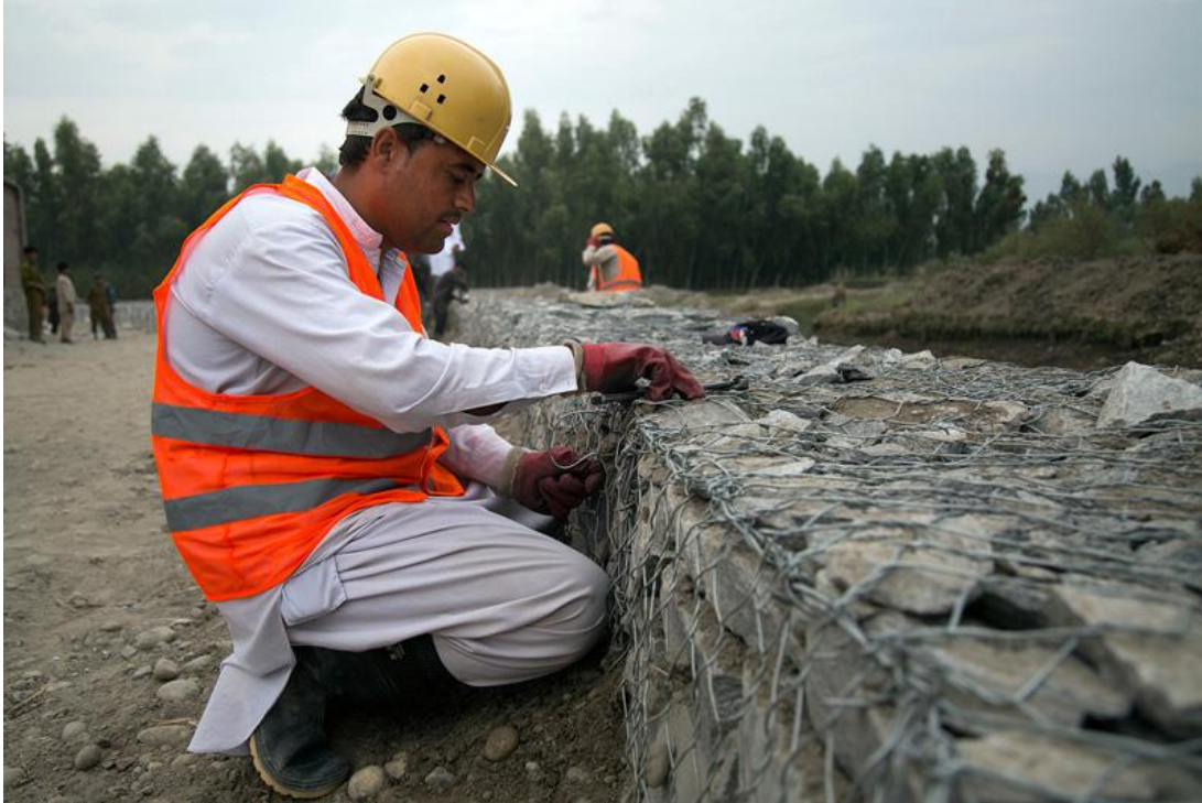
IOM completes flood protection walls in Afghanistan's Nangarhar, Kunar provinces. Photo: IOM
