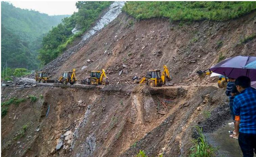
Imphal: Repair works underway National Highway No. 37 after a landslide triggered by heavy rainfall near Imphal on Thursday, June 14, 2018. (PTI Photo)
