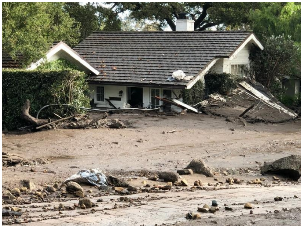
Montecito, California, flood and mudslides damage, January 2018. Credit: Santa Barbara
