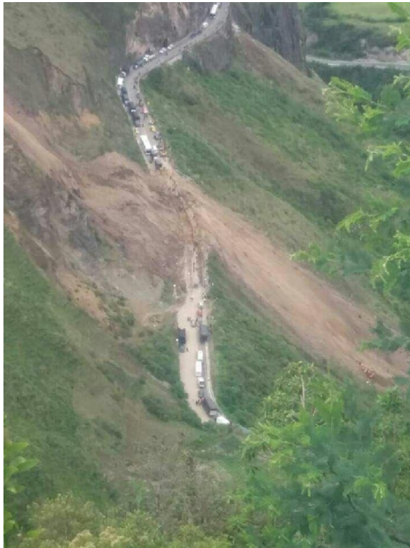
(on left) Scene of the landslide near Mallama, Narino, Colombia, January 2018. Photo: Dirección Nacional de Bomberos de Colombia del Ministerio del Interior.
