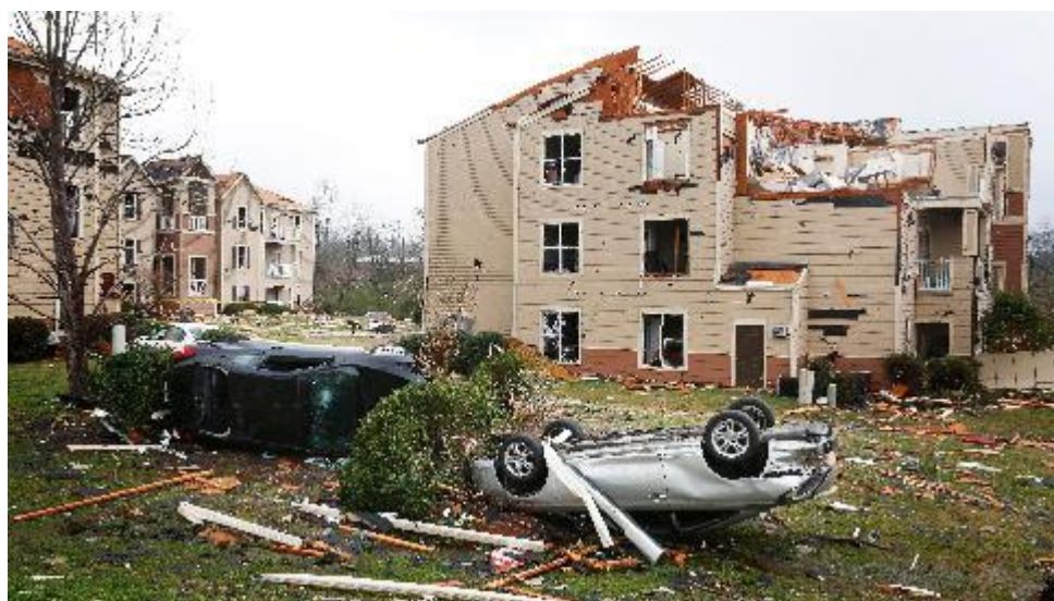
Two cars are turned over in front of a tornado-damaged apartment complex in Jacksonville, Alabama. (AP Photo/Brynn Anderson)
